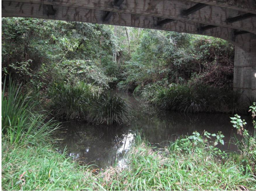
Plate 5: Stony Creek under existing Pacific Highway
