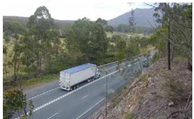
Existing Pacific Highway constrained between cutting and Main Northern Railway line
