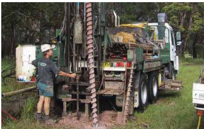
Borehole drilling for geotechnical investigation
