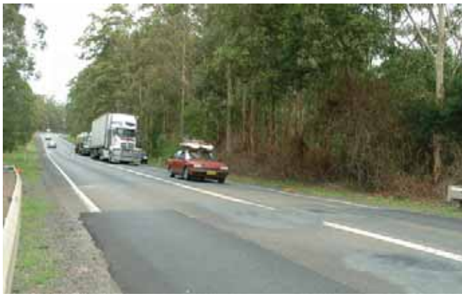
Existing Pacific Highway at Stony Creek
