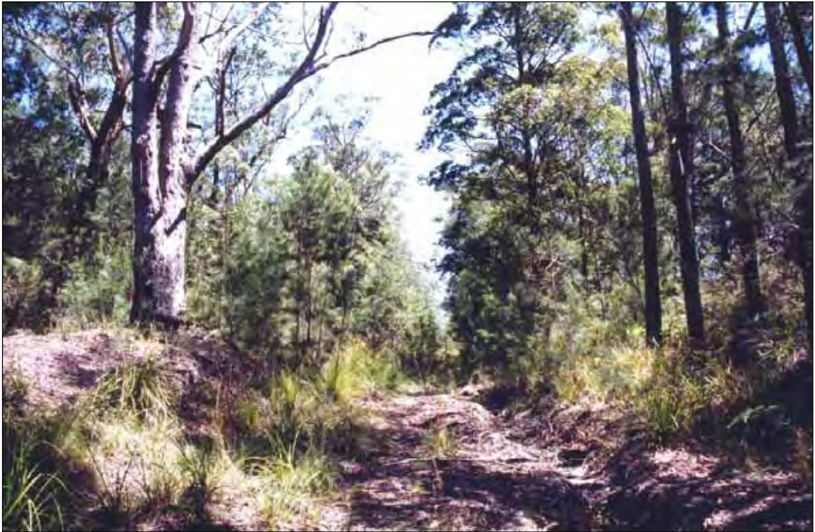
Plate 12: Site H23 - section of a former Pacific Highway alignment dating to the 1940s, looking south.
