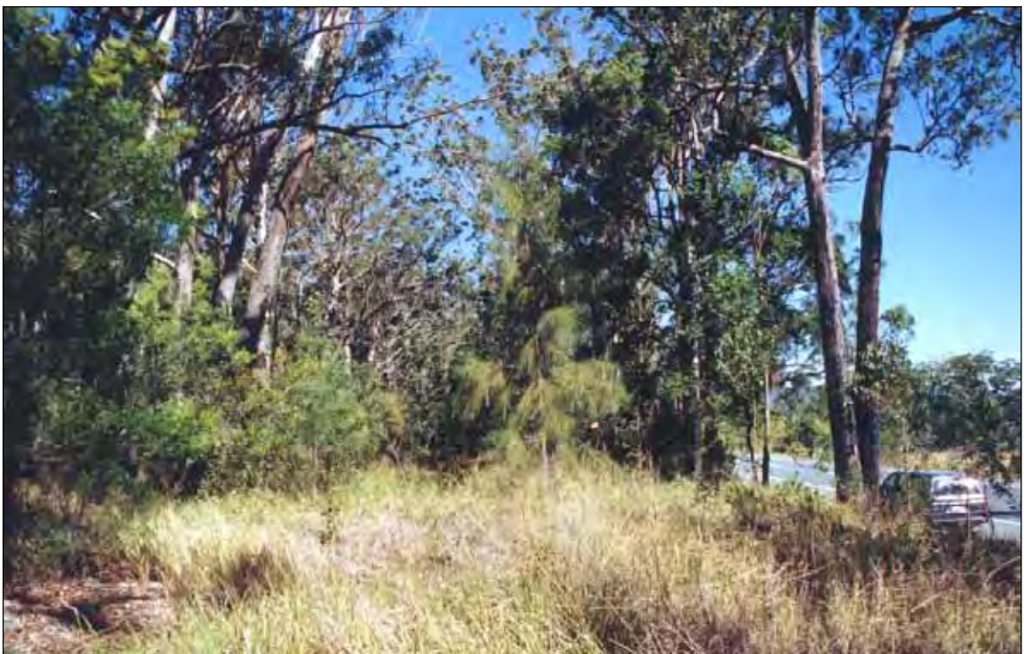
Plate 15: The northern end of site H32, a remnant section of former Pacific Highway alignment, looking south.
