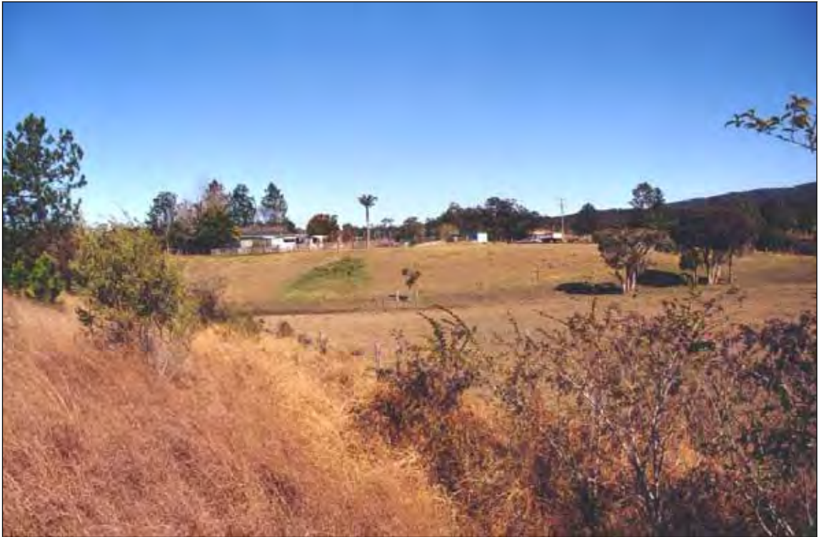
Plate 8: General view of PAD5 – the elevated terrace and associated basal slopes in middle distance – looking southwest from existing road embankment
