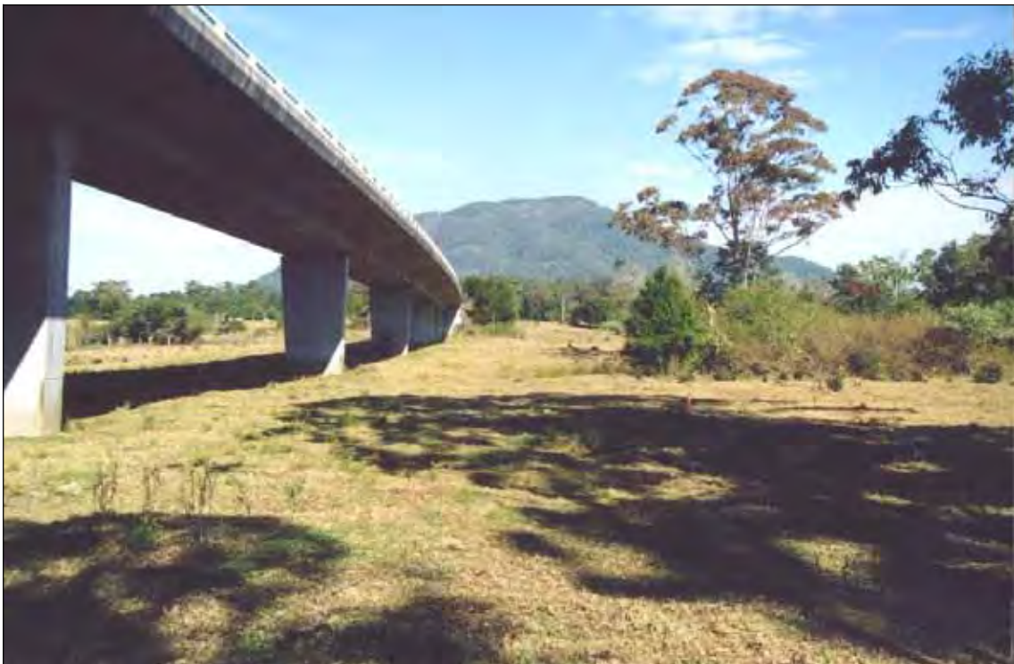
Plate 5: Location of PAD2 (are to right of bridge spans) – looking southwest towards South Brother Mountain.
