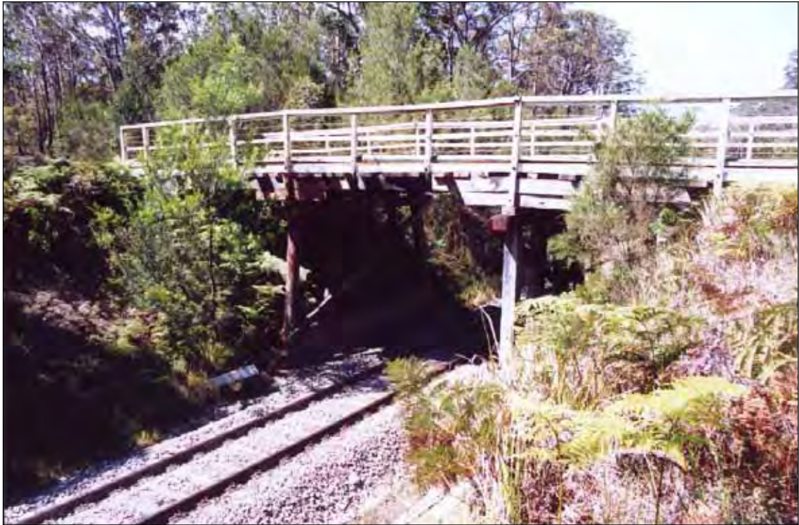
Plate 10: Site H30 - wooden rail bridge near Stewarts River – looking northeast.
